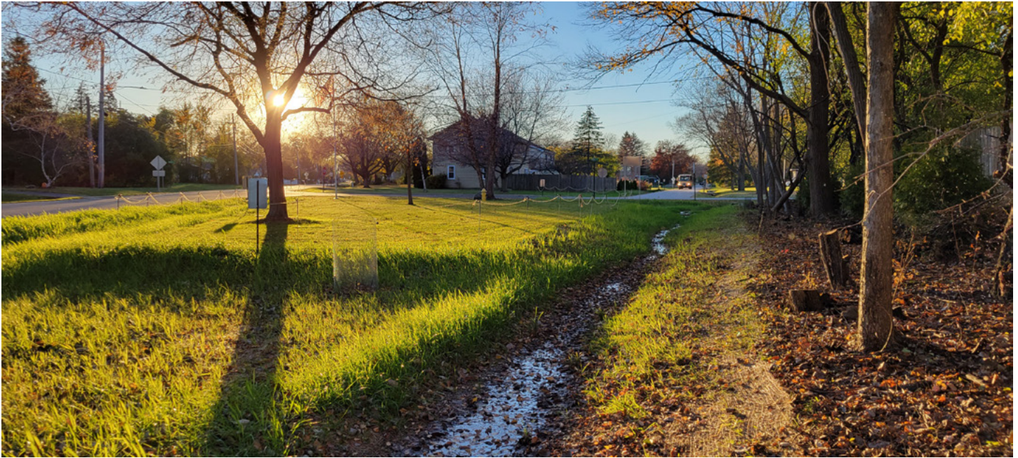
Plants started growing immediately in the ditch's matting, and the ditch now mitigates soil erosion and controls sediment.
