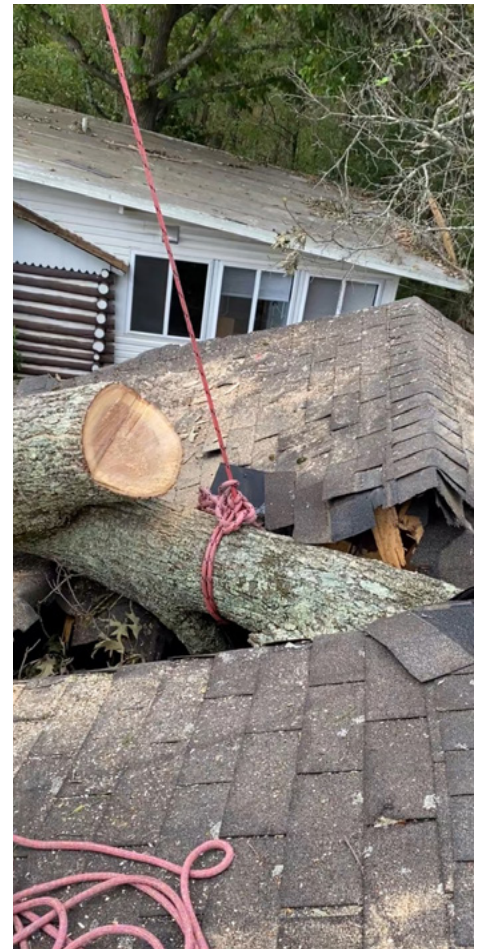
The stem of a large red oak is being removed by a crane. The oak fell on a house during Hurricane Helene. Photo by April Wilson, Stump Sprouts Tree Consulting.
